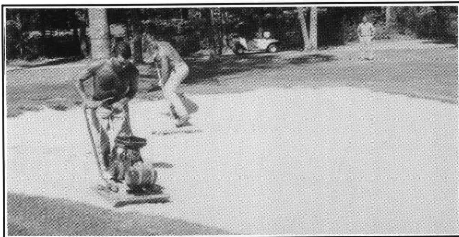
TOUGH WORK — These two able-bodied men, Scott Listul in the foreground, and Riley Kiefer utilize a Wacky Packer and rake to firm up the Ohio Best sand.
