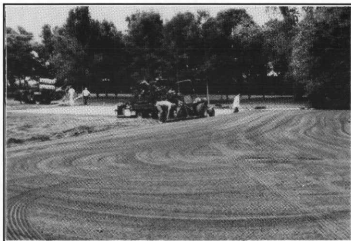
Putting finish grade on the tee.
