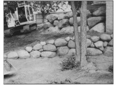
place. The drain tile can now be installed behind the first tier and the fabric. It is vital to remember to compact the soil thoroughly behind each tier as you go. This is extremely important.
