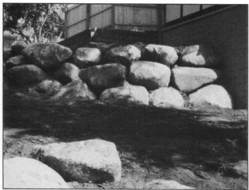
Boulder walls will provide good soil retaining strength and provide a look that golfers will love. The expense of a boulder wall is not much more than that of a properly constructed timber wall, and usually cheaper than prefab or "keystone" walls. Considering how long it will last, the extra cost of a stone wall is worth the extra expense over a wood wall.
