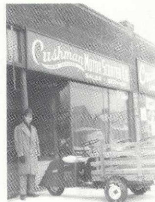
Our Original Location in 1949 3205 Cedar Ave., Minneapolis
