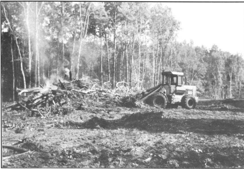
CLEARING AND GRUBBING a year ago on the fifth hole.
