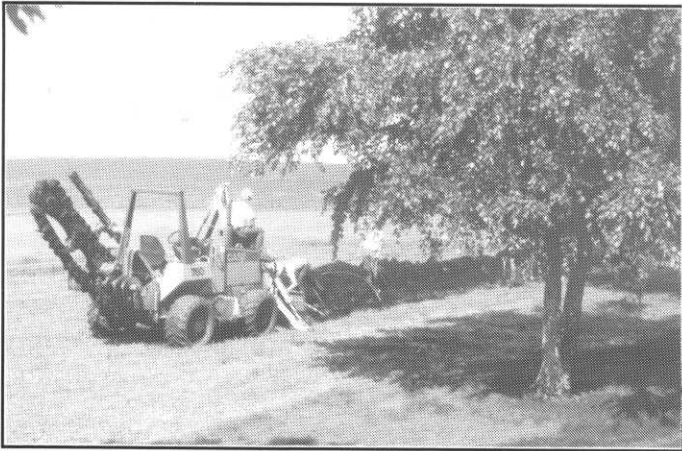
Laying cable and power lines to the Corporate Village
