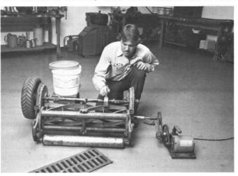
Use of a backlapping machine (lower right) allows the reel of a wheel friction driven mower to rotate backwards. A reel sharpening compound should be applied across the entire width of the blades while they are rotating.
