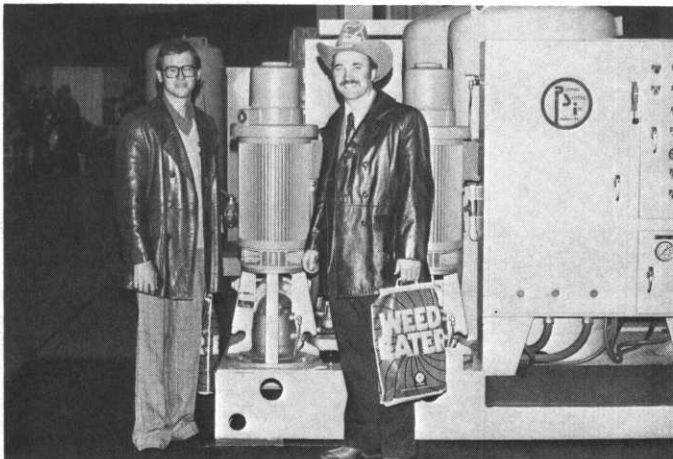
PARTNERS. Dale Hendrickson and Leif Erickson check out the pumps.
