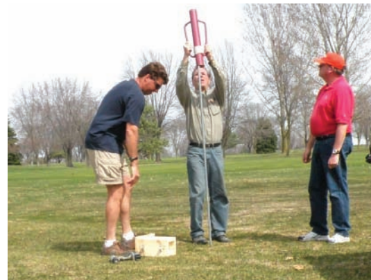
Installation of the posts.
