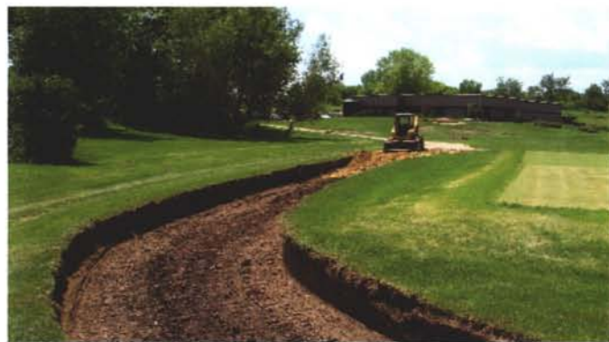
Constructing the access road to the bridge
