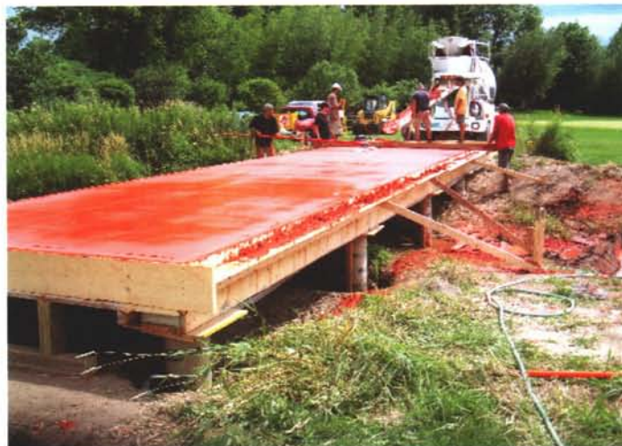
Pouring the concrete deck
