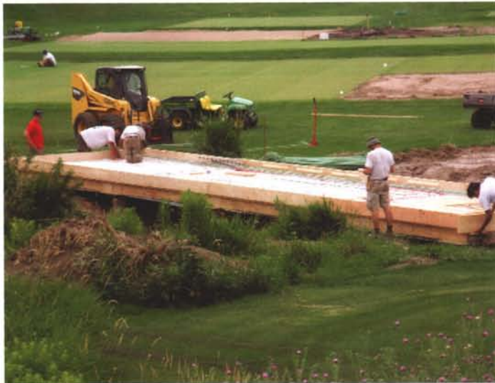
Building the forms for the concrete deck
