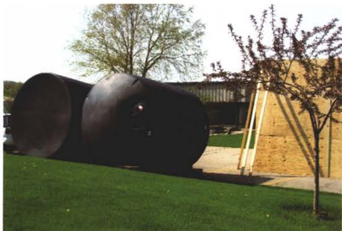
Two 4,000 gallon rain barrels that will be used to store rainwater to irrigate the Noer Facility front lawn.
