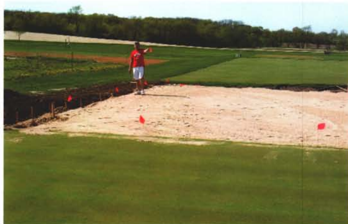
Turf student Bill Kreuser puts the finishing touches on his newly constructed USGA Green.
