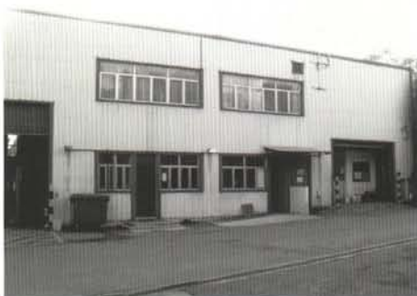
Grounds maintenance building.
