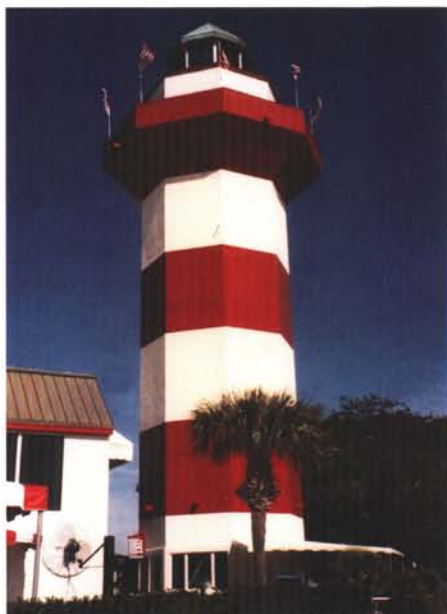
The lighthouse at Harbor Town overlooks the 18th hole, a golf course designed by Pete Dye and Jack Nicklaus.
