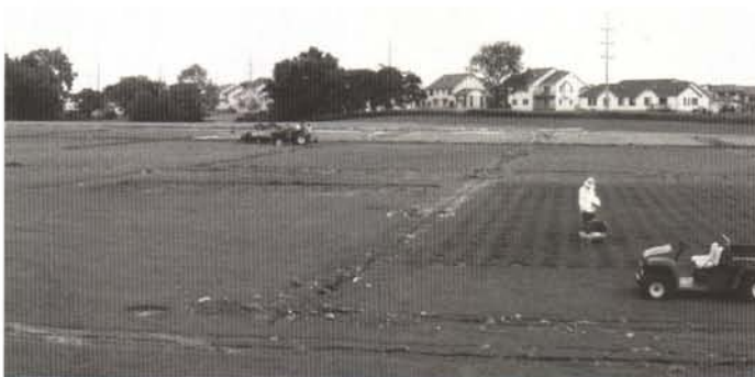
The staff makes connections while the "Toro Dingo" trenches ahead.
