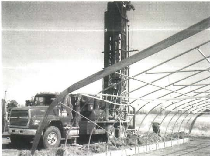
Drilling the new well.
