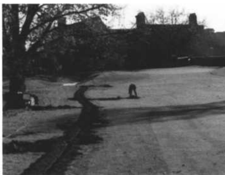
Triple row irrigation installation.
