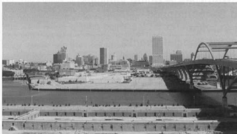
The Milwaukee skyline from a top the concrete storage bins at MMSD on Jones Island.
