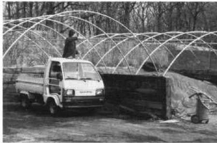
Support pipes are tightened.
