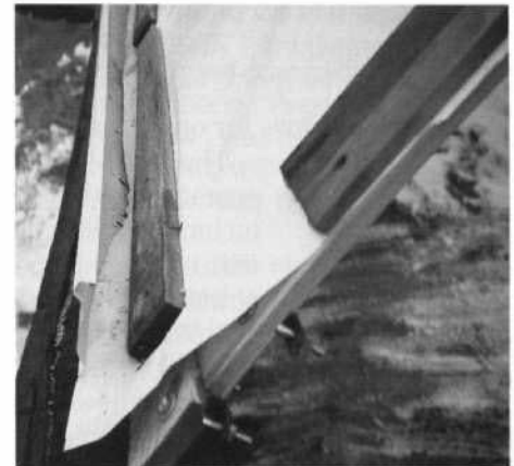
Plastic is positioned between the boards and screwed together.
