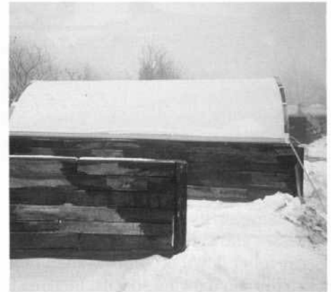
Rain never entered the open ends of the bins.
