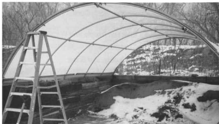
The front and back are left open. This allows the wind to blow through the structure
