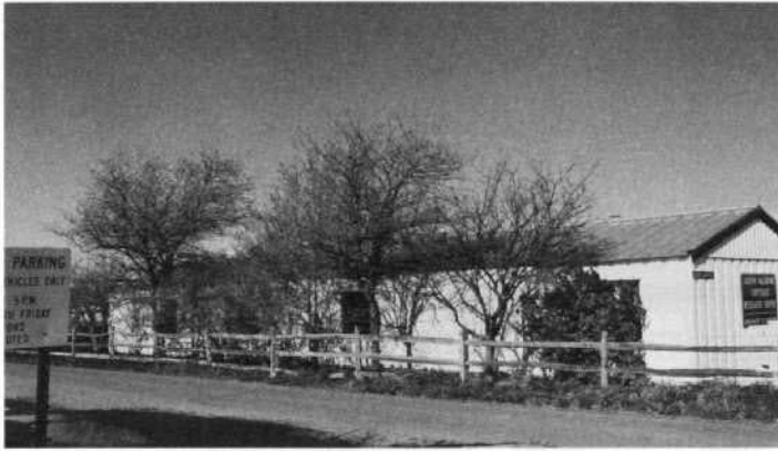
Headquarters building of the Joseph Valentine Turfgrass Research Center.
