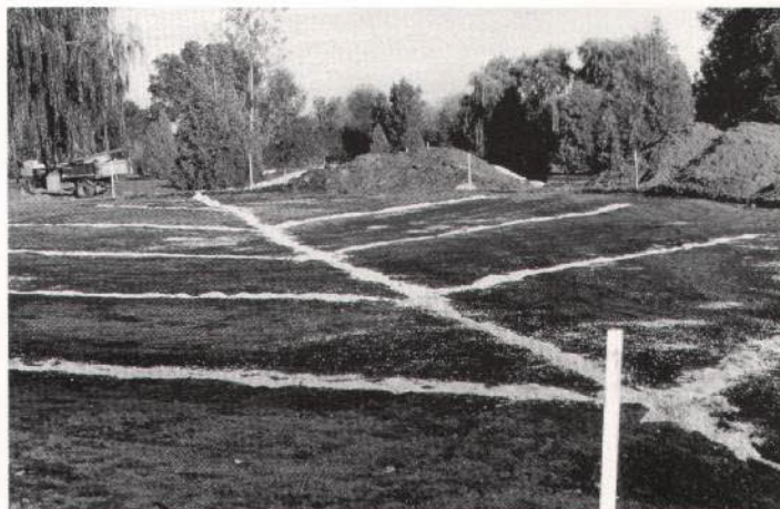
Installing Drainage.
