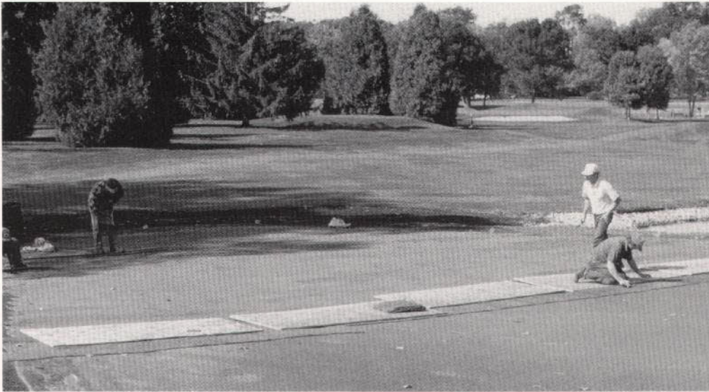
Careful alignment of the sod to lessen seams.
