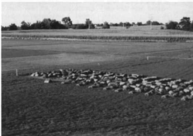
Figure 3. Sod is stripped away from the future site of organic amendment evaluation green.
