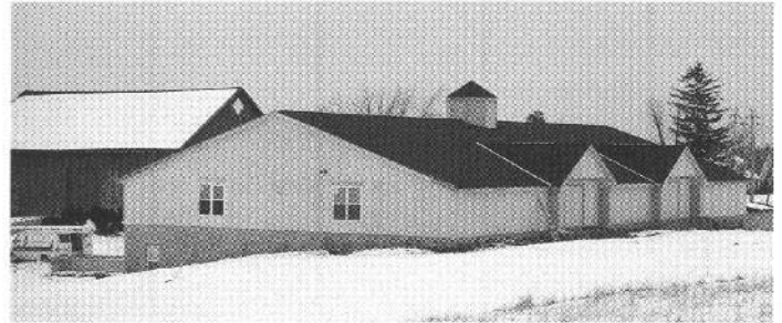
Bob Erdahl's new building at North Shore reflects its very urban setting and concomitant zoning requirements. It is flanked by the barn it replaces and also some very expensive homes. This shop looks like a very nice stable. I like to call this beautiful building "the Yuppie Shop" (because of its appearance, not Erdahl's status!)
