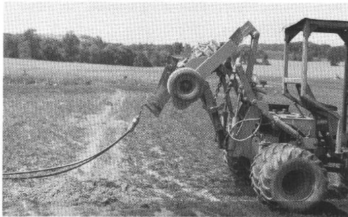
Two pieces of 1" poly pipe were pulled in tandem for adjoining plots.
