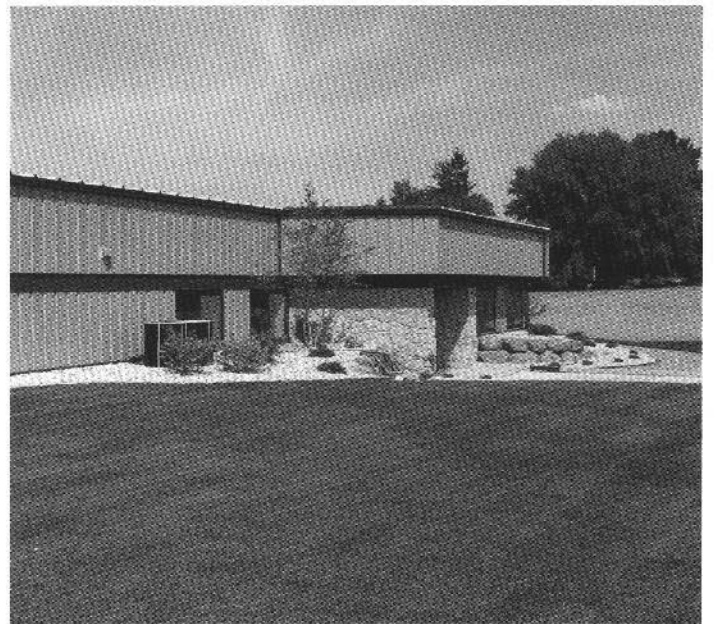
The front entrance, looking east to where the old buildings once stood.
