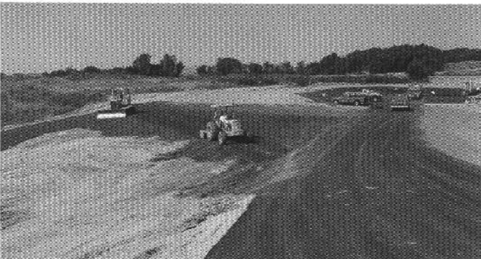
Black silt loam soil was spread over the fill where the old buildings were only days previous.
