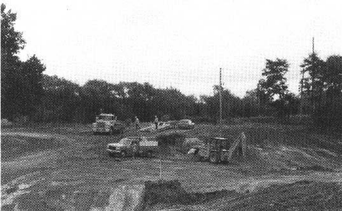
An underground fuel tank was removed "by the book, to the letter".
