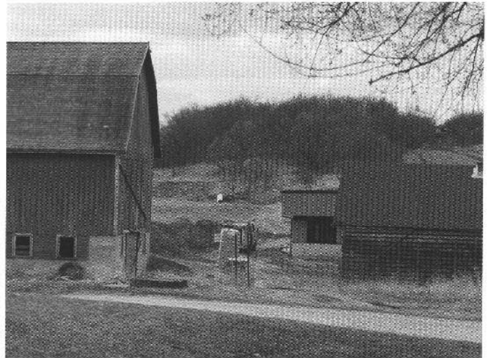
A look at the NOER building through the old farmstead.
