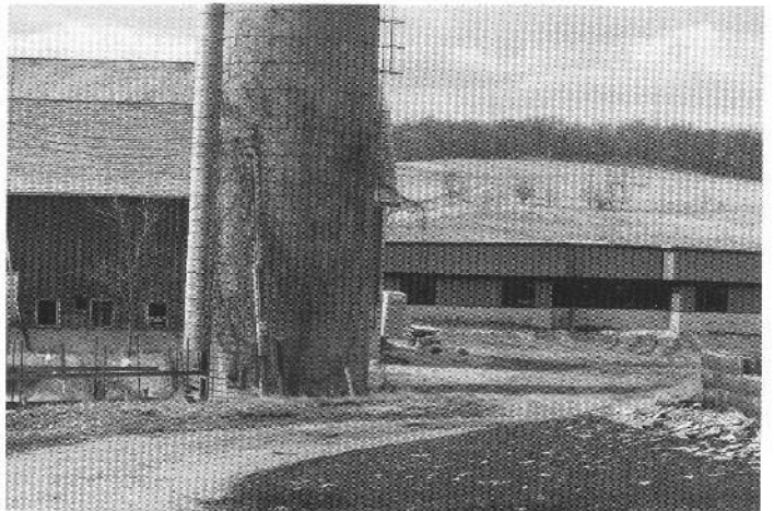
Another look at the mess prior to demolition.
