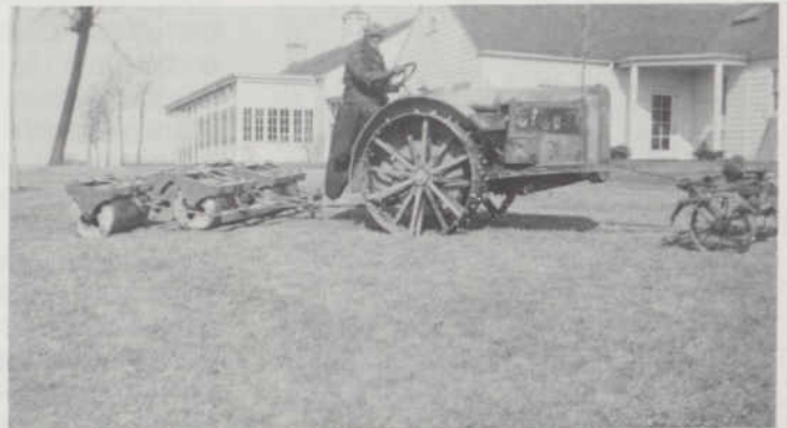
Frank during construction at Ozaukee Country Club.
