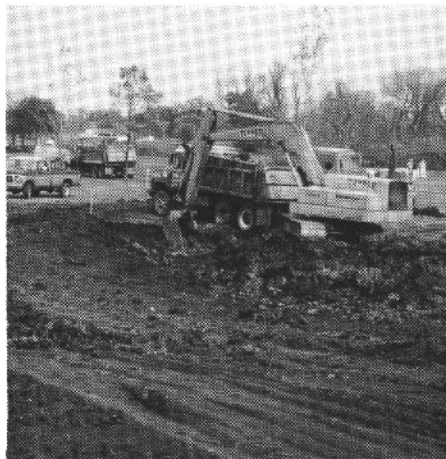
Pond excavation — from plans to the field.
