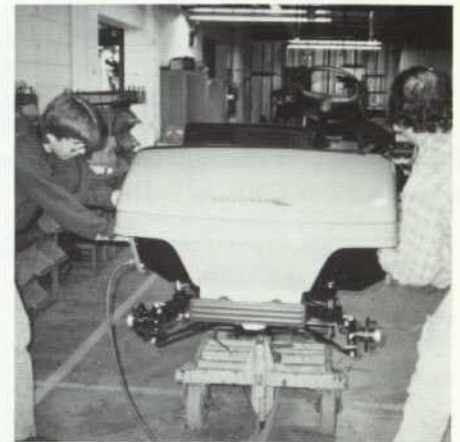
Vehicle controls are being installed here.
