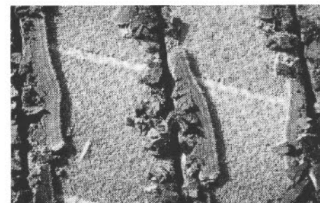
Various stages of the grooving process.
