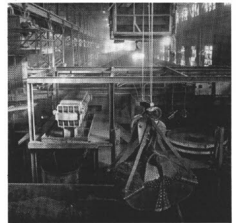
Milorganite storage barn.
