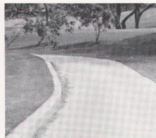
Curbed cart path.
