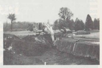
ously pumped from the pond site for visability and workability. The bottom and banks were carefully shaped to conform to the architects and D.N.R. specifications. This portion of the construction took about a week to accomplish.
