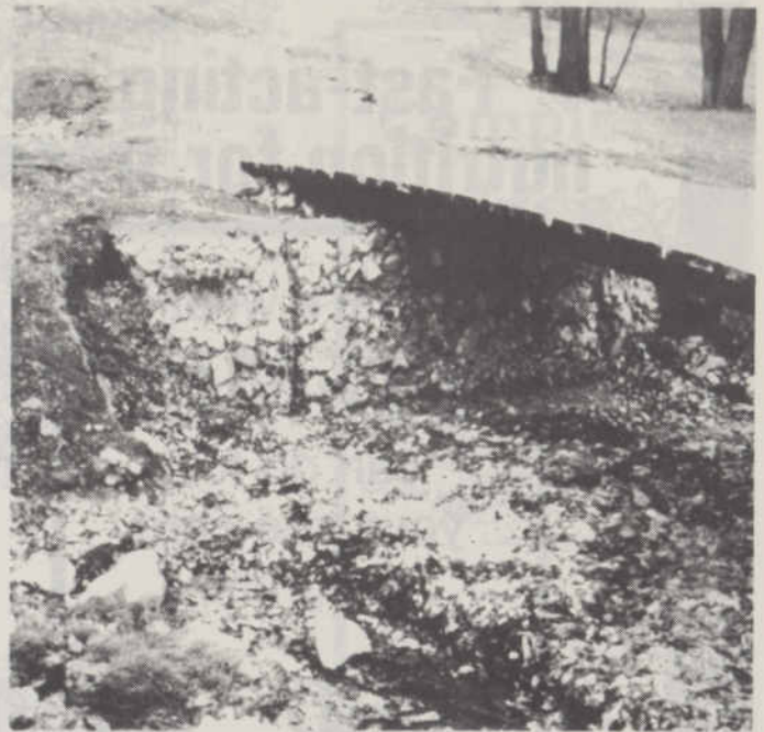
Rock-filled gabions in place.
