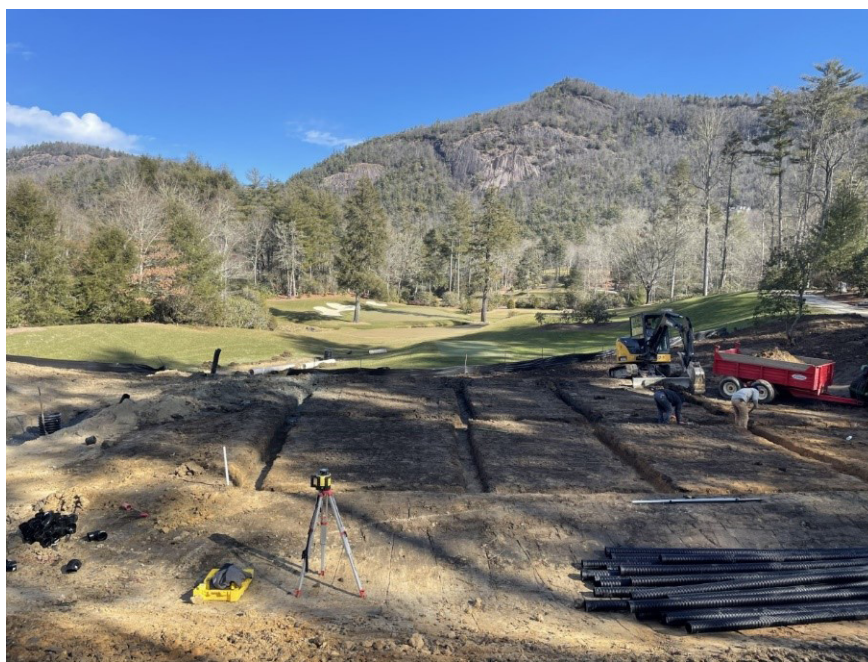
New tees on number 17, the signature hole with its towering eastern hemlocks and Chimney Top Mountain in the distance, with the trenches dug for drainage to be installed later that day.
