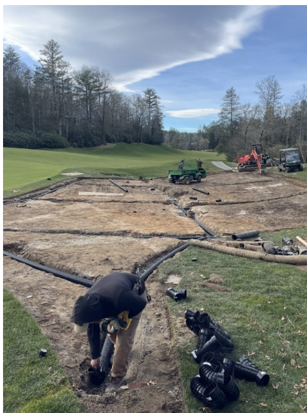
Installation of drainage tile on the left side of number 10 primary rough next to a roll off area by the green, which has drainage issues.
