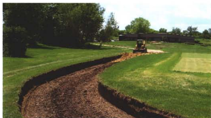
Constructing the access road to the bridge
