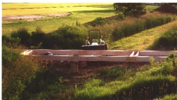
Forms were constructed for pouring the concrete piers and deck support beams
