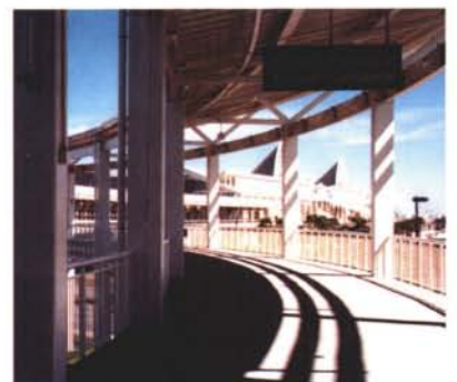
The new addition to the OCC is huge beyond words.
