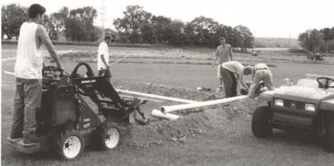
Plant pathology graduate students conduct their work while the irrigation system goes in around them.
