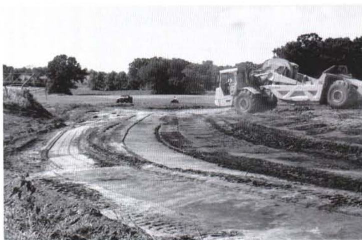
Bruce Company reshaping new 10 acres.
