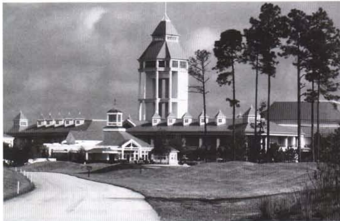
A ride in an elevator takes you to the top of this observation town and affords views...
