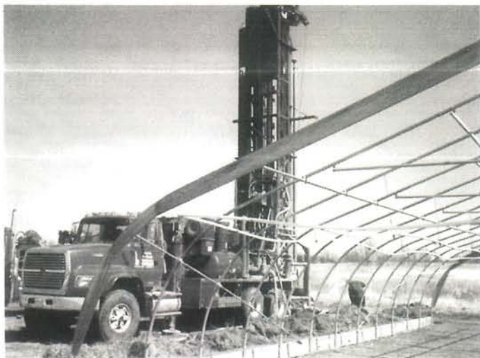
Drilling the new well.
