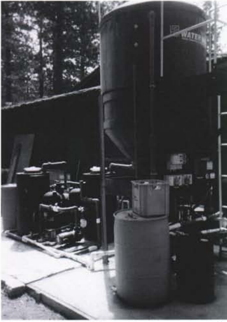
A water clarifier is used to remove sediment and pollutants from wash pad water to prevent discharge into Lake Tahoe.
