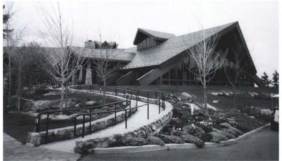
The clubhouse at Edgewood GC is extensively landscaped. By mid-May, the deciduous trees still did not have leaves due to the cool climate.
