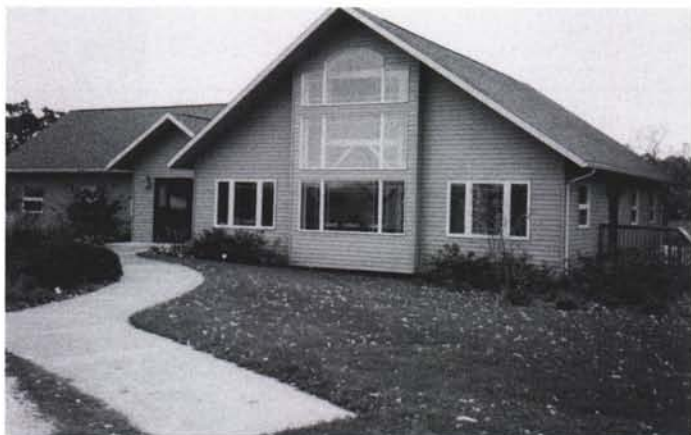
SSE headquarters building, located above the farmstead. This is a front view.
