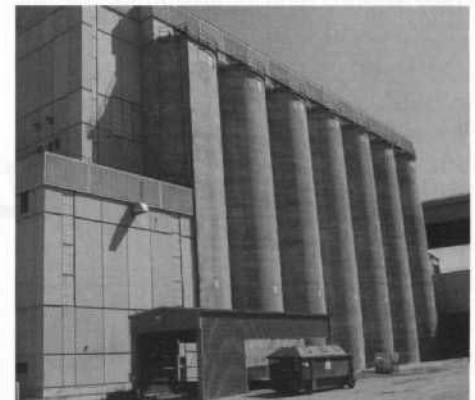
Massive storage bins, part of the new Milorganite facility, hold millions of pounds of America's favorite natural organic fertilizer.
