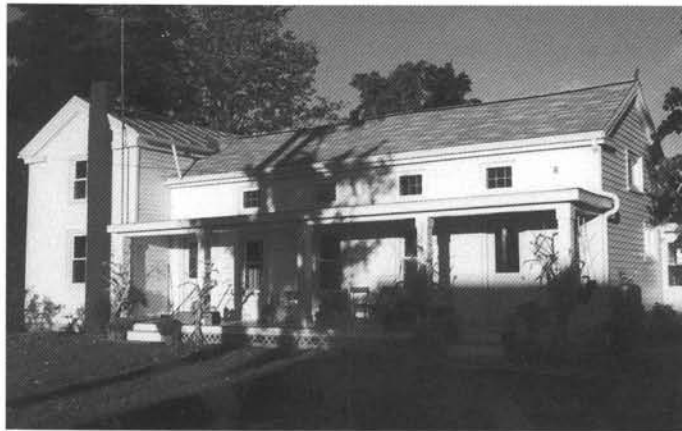
The remodeled farm house the Rossi's now call home.
