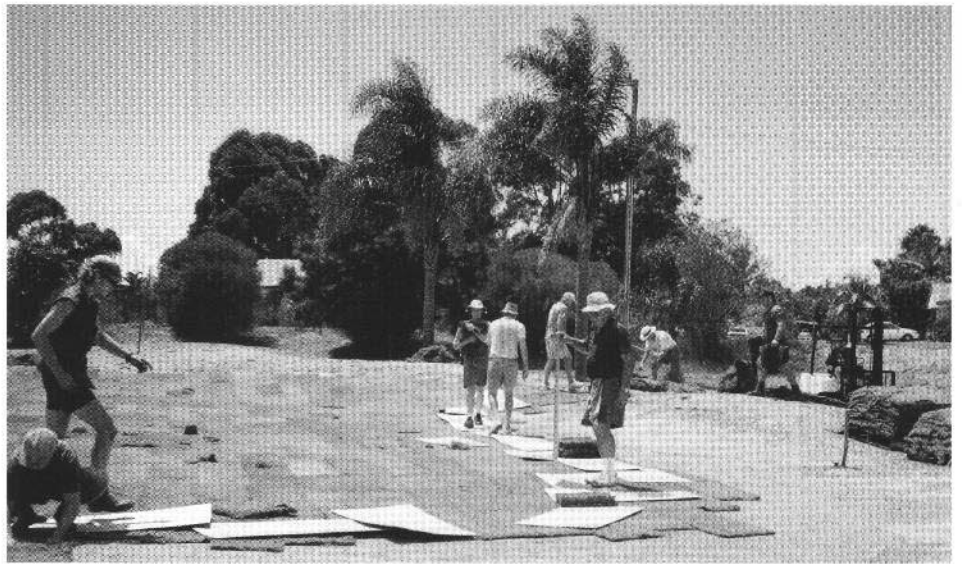
Reconstruction of a green at Southport CC on the Gold Coast south of Brisbane. The grass type is 328 Bermuda which is commonly used on greens in the region. The man with the white hat is the green committee chairman!
