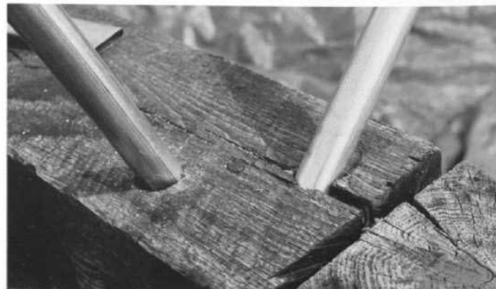
Pipes are positioned into the pre-drilled anchor holes.
