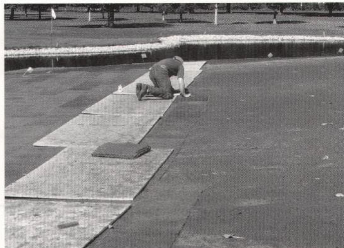
The Sod Process — plywood over the new sod never disturbing the prepared greens mix.
