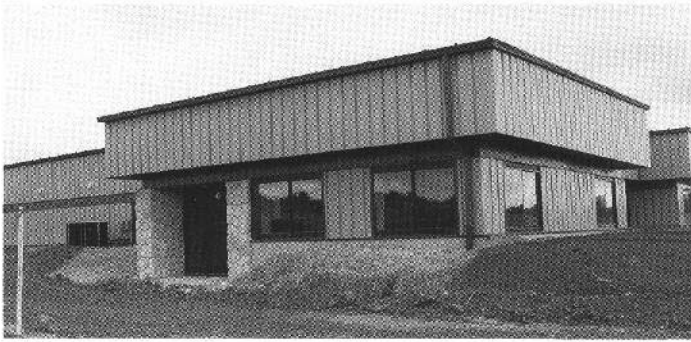
Early stages of landscaping at the building entrance.
