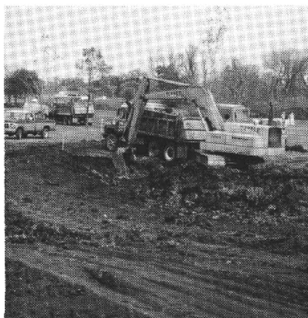
Pond excavation — from plans to the field.
